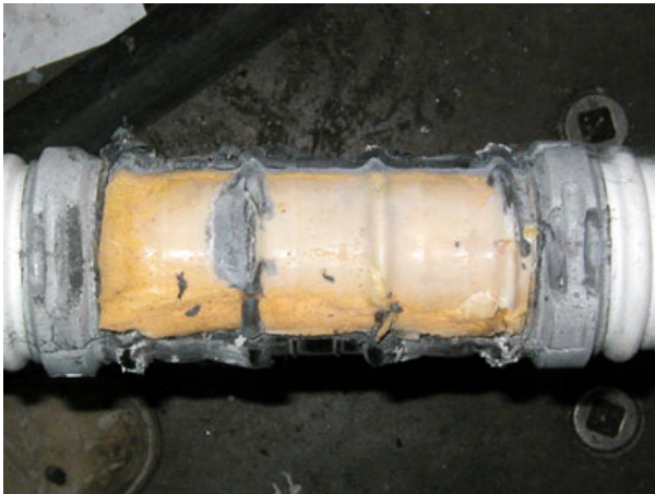
(c) Sponge after grouting
