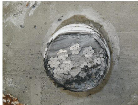
(b) Concrete block
