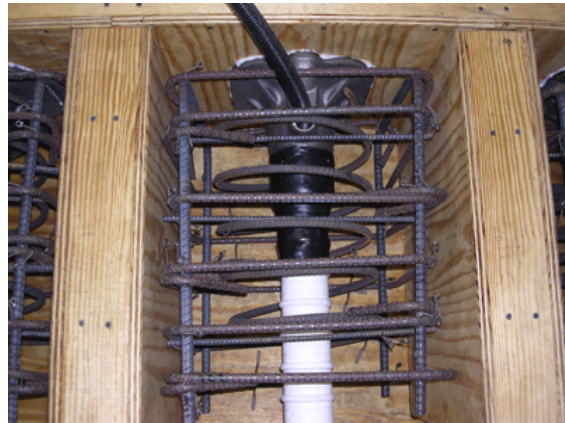
(b) Anchor plate within reinforcement
