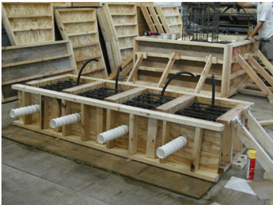
(c) Concrete form
