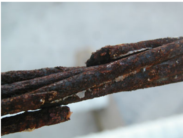
(a) Fractured wires
