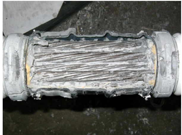
(d) Strands after removal of sponge and grout
